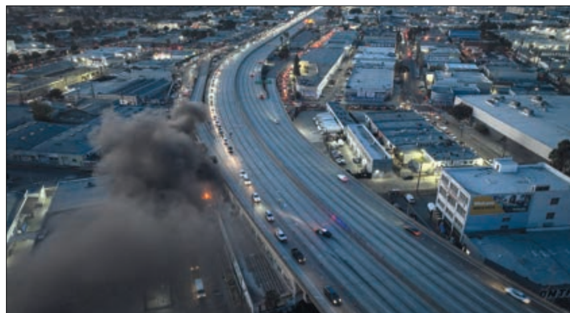
LOS ANGELES — Still surreal — the continuing visions of an empty freeway in the middle of LA: Smoke rises from a small fire as motorists exit through a ramp off Interstate 10, where a section of the freeway is closed due to a recent fire in Los Angeles, Tuesday, Nov. 14, 2023. It will take at least three weeks to repair the freeway damaged in an unrelated arson fire, the California governor said Tuesday, leaving the city already accustomed to soul-crushing traffic without part of a vital artery that serves hundreds of thousands of people daily.
