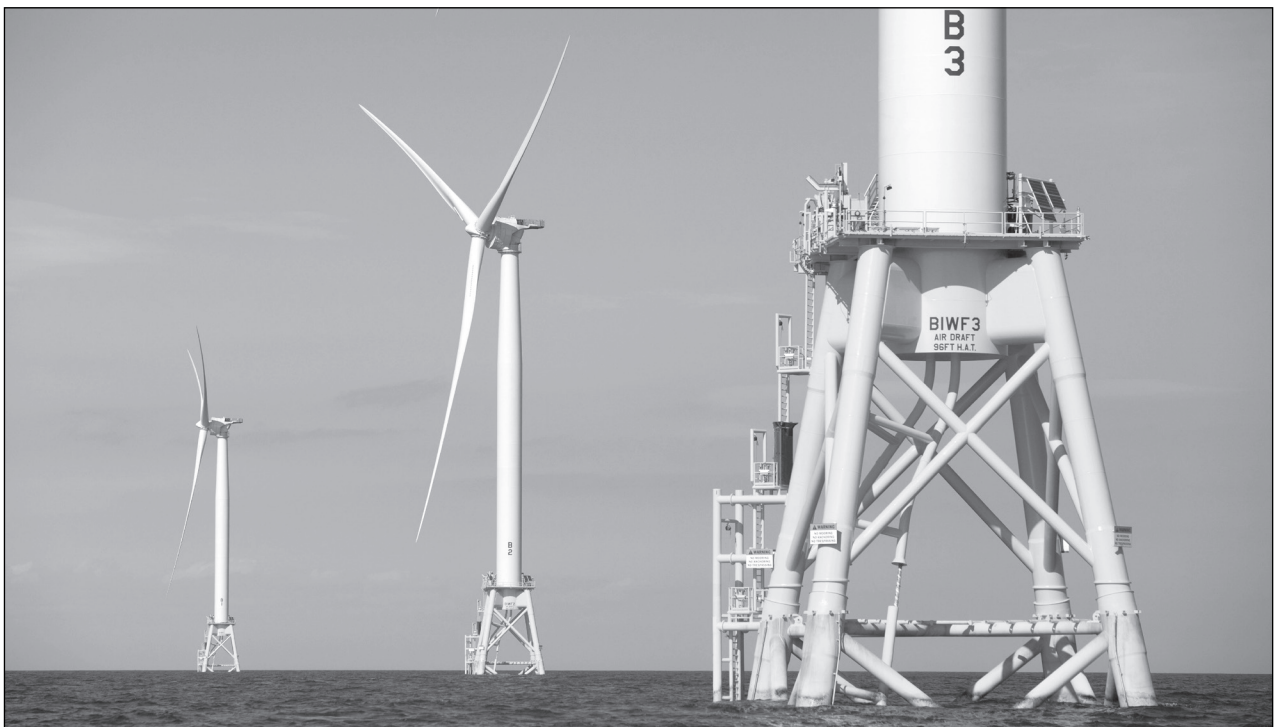
Three wind turbines stand in the water off Block Island, R.I., the nation's first offshore wind farm AP Photo/Michael Dwyer, File
